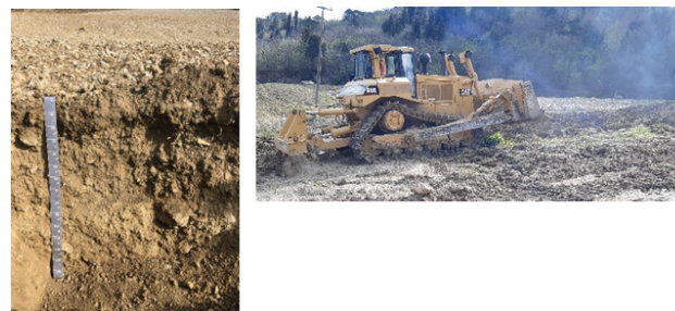
Figure 5 Soil profile dug after land preparation for vineyard plantation. The topsoil (0-30 cm) was removed, then the subsoil was deep ploughed (30-90 cm) and mixed by excavator and then land levelled. After all, the topsoil was replaced.
